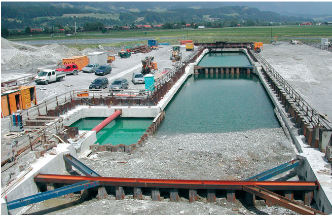
Analyzed with DC-Software Sheet pile walls at the Brenner base tunnel (Brixlegg)
