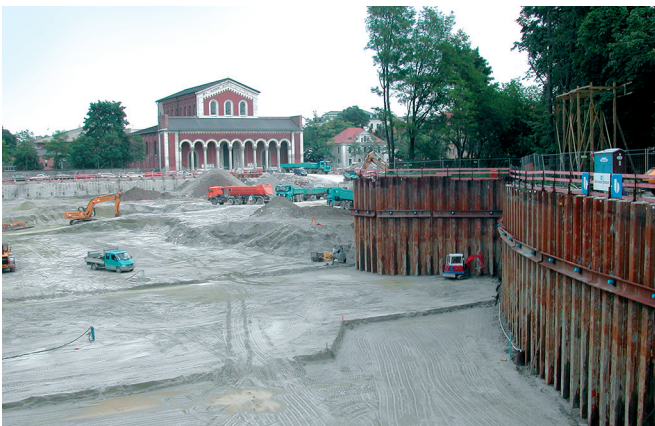
Analyzed with DC-Software Sheet pile walls at the Lenbach gardens in Munich
