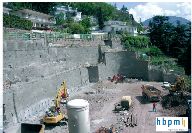
Analyzed with DC-Software Multi-step nail wall in Bolzano
