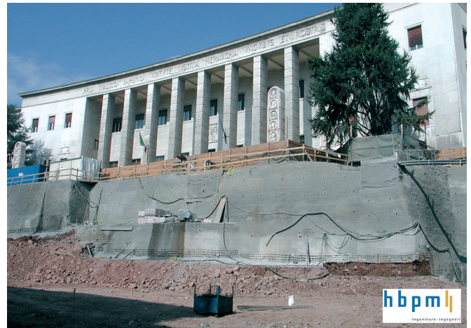
Nail wall at the court building in Bolzano
