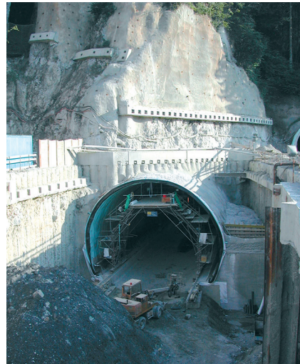
Analyzed with DC-Software Bore pile and nail walls at the Brenner base tunnel (Brixlegg)
